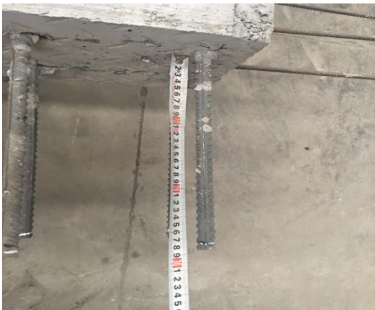
套筒钢筋过长需切割
