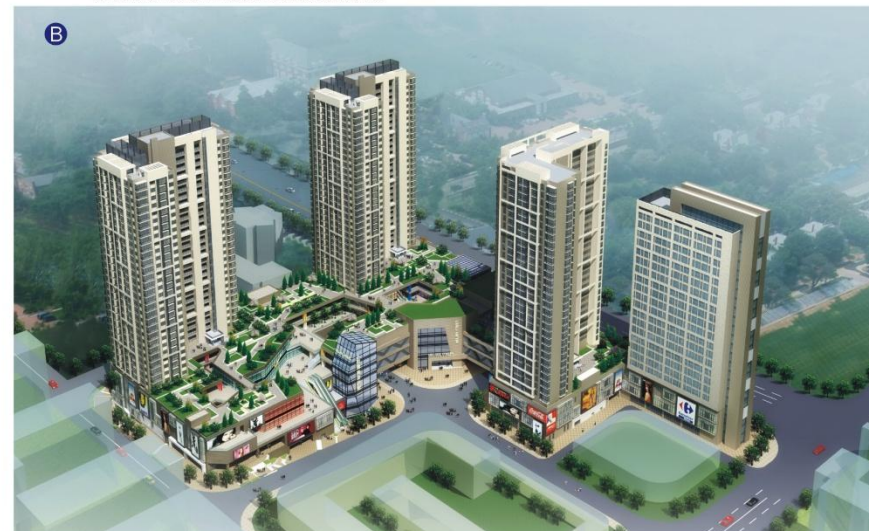
A 荆州楚天都市郎园 Jingzhou Chutian City Park 建筑面积: 96000M 2 结构层次: 框剪结构, 地上33层 所获荣誉: 国家AAA级文明工地 Construction area: 96000 square meters Structure level: frame shear structure, 33 floors on the ground Achievements: National AAA-class Civilized Standardization Site
