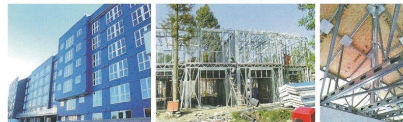
薄壁钢结构多层住宅 Multi-floor housing with light-gauge steel structure
